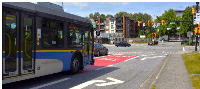
The bus lane along Keith Rd is supported by red paint, a right-turn pocket, and a left-turn restriction at the intersection with Bewicke Ave.
