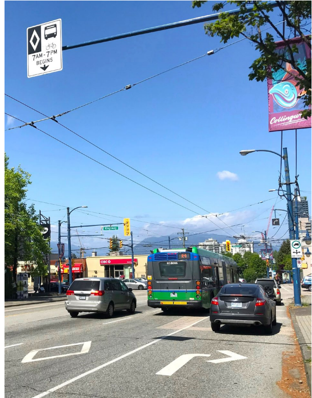
The approach lane on Joyce St at Kingsway is supported by a right-turn pocket. Parking was removed to lengthen this pocket and minimize friction with buses. The project reduced average travel times by more than 30% all day.
