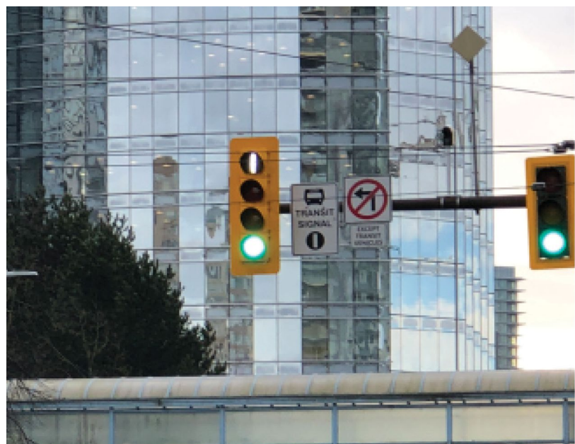
Bus-only signal at Metrotown.
