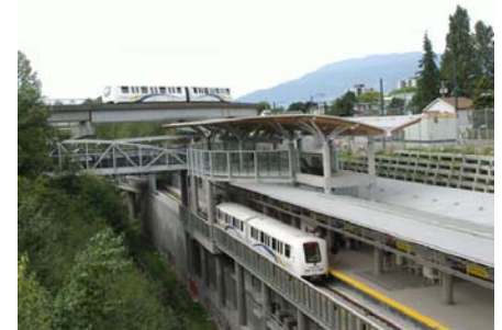
Commercial Drive SkyTrain station is part of the major transit hub at Broadway and Commercial
