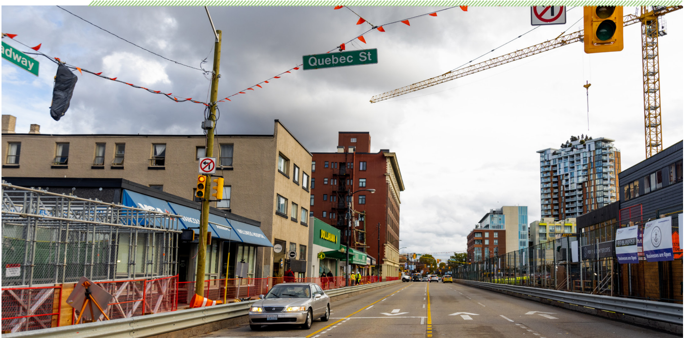
Source: Broadway Subway Project
