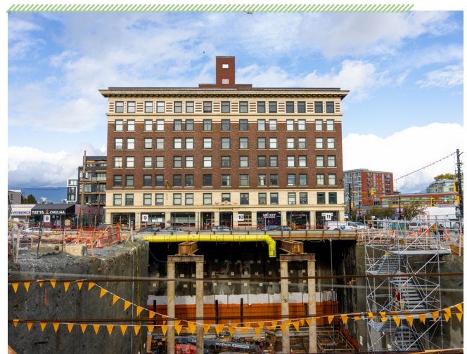
Source: Broadway Subway Project
