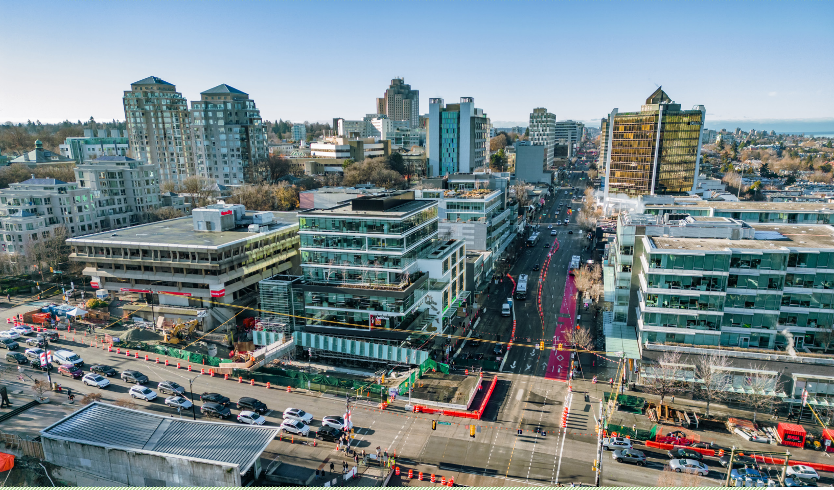
Source: Broadway Subway Project
